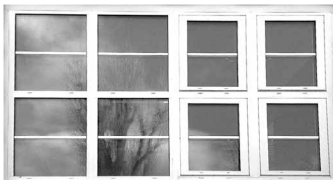
Photo 3. ALUFIRE fire resistant technical window with a fixed wall (intra-glazing dividers)
