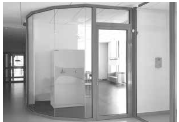
Photo 1. The above example of angle wall is an alternative for expensive constructions with bent glass. An additional value of such a solution is no deformation of the image when compared to the bent glass.
